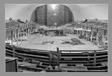
**Top**: New steel beams reinforce the floor underneath the organ. Re-winding of the organ is underway. Photo courtesy of Rocky Mountain Organ Co.
