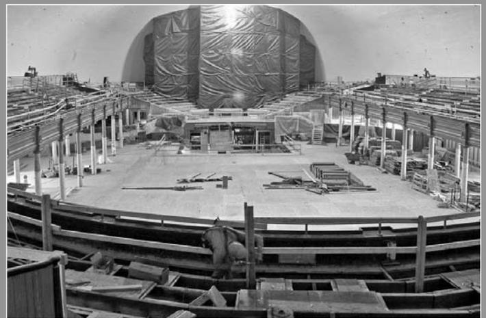
**Top:** New steel beams reinforce the floor underneath the organ.
