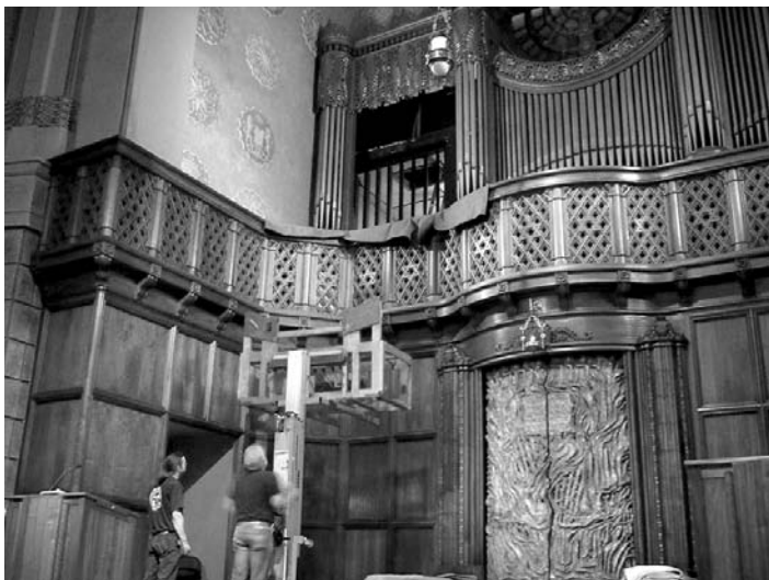
Left: View of the Temple front during removal of the organ.
