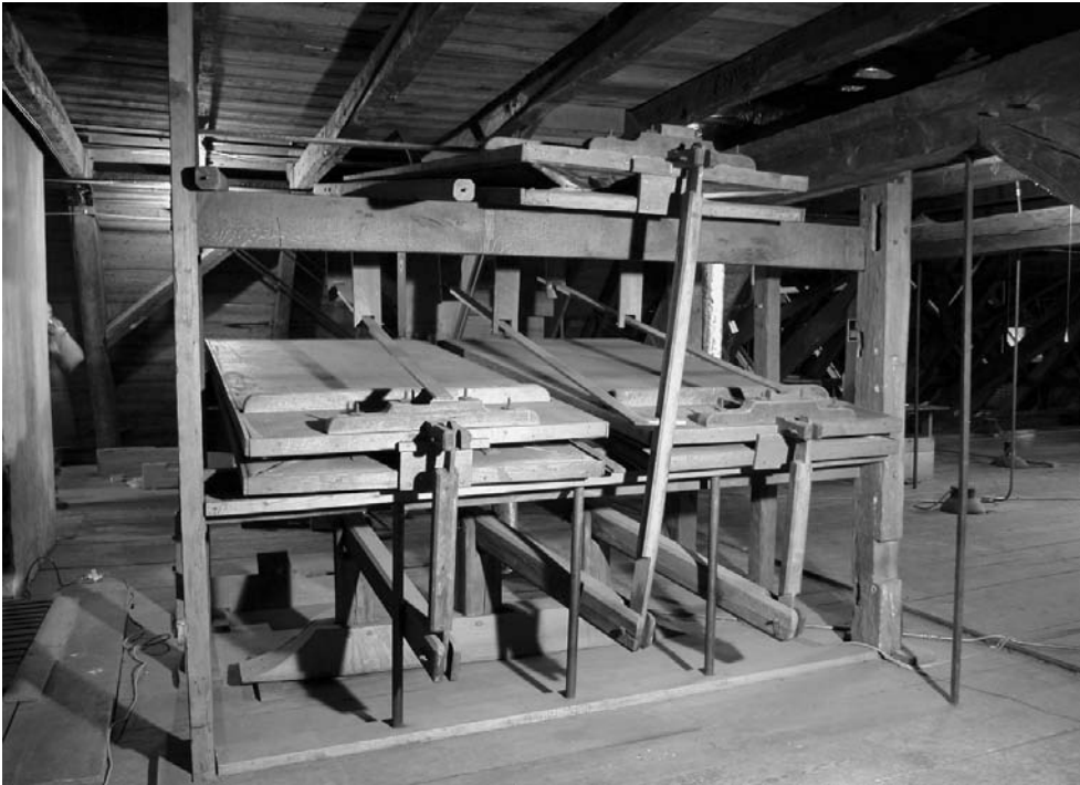
Left: Bellows in Home Church attic.
